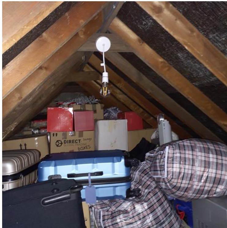
Photo 13. Main roof void.
