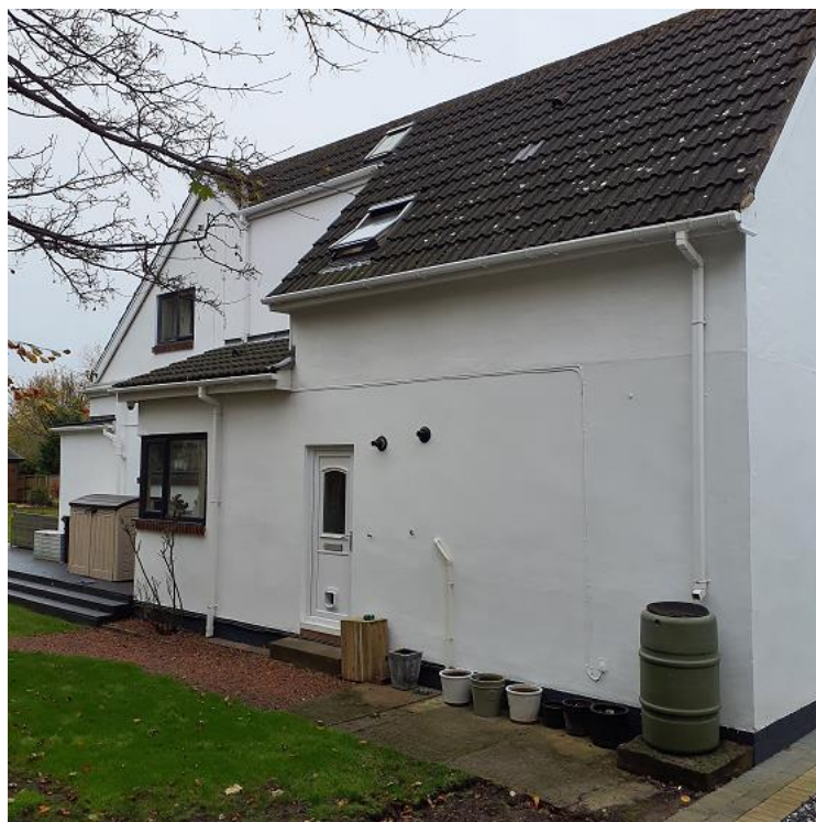
Photo 2. Building viewed from the NE
