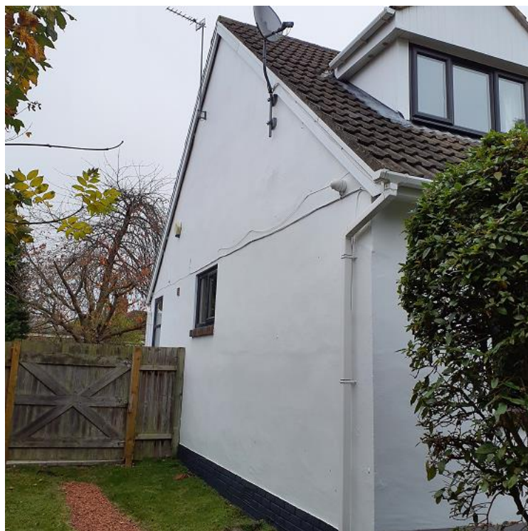
Photo 4. Building viewed from the SW.
