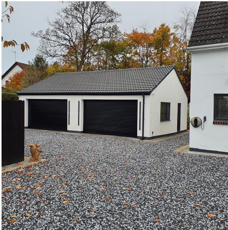
Photo 5. Garage viewed from the SW.
